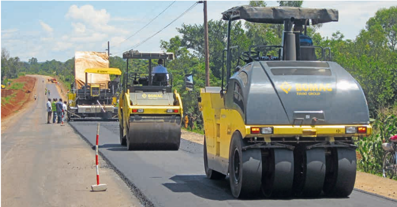
The BOMAG BW 24 RH rolling asphalt in Uganda.
